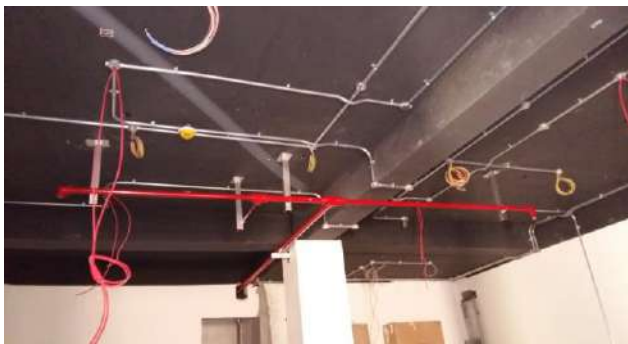
Maintenances & Renovation work - Novac 1230
