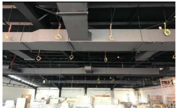
Maintenances & Renovation work - WARE HOUSE AT DUQM
