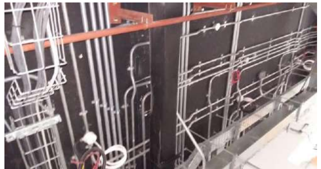
Maintenances & Renovation work - Electrical conduiting & trunking works at NBO H.O.
