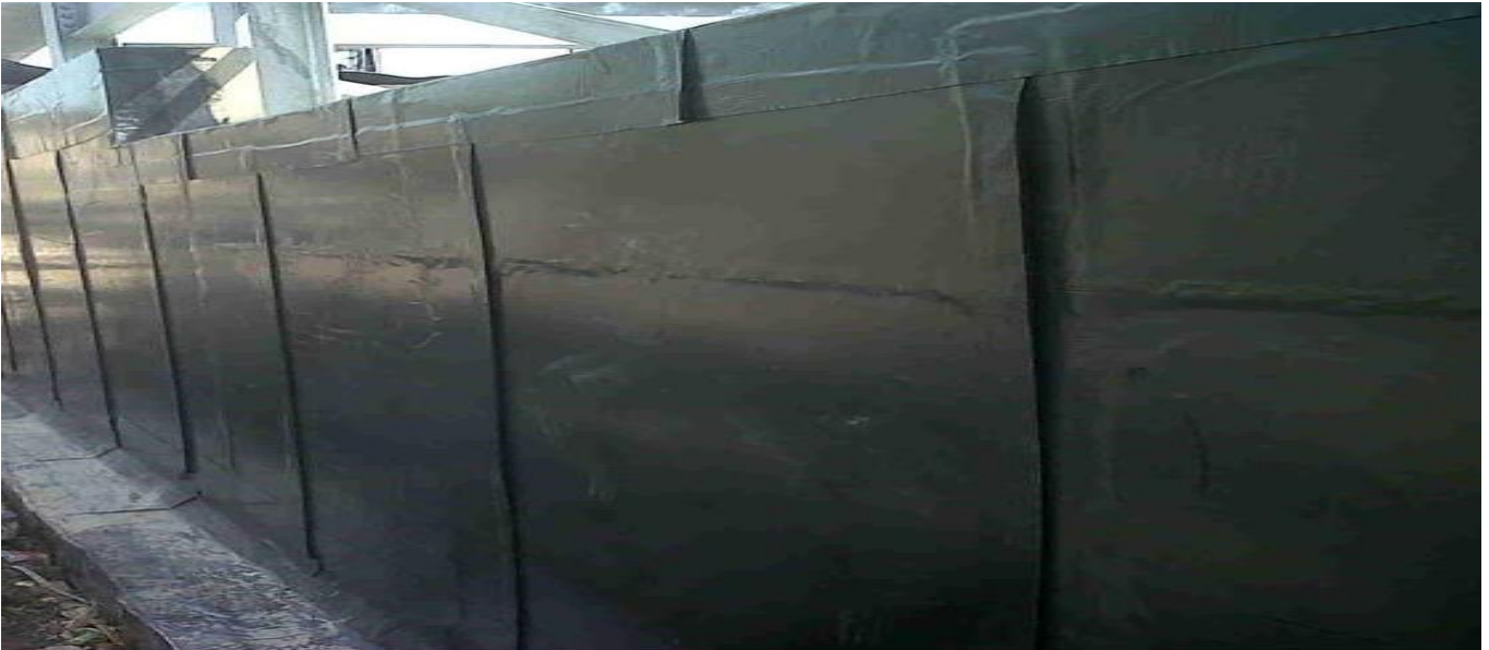
Self-Adhesive membrane work @ RGF Water Tank Thoshiba Site – Sohar
