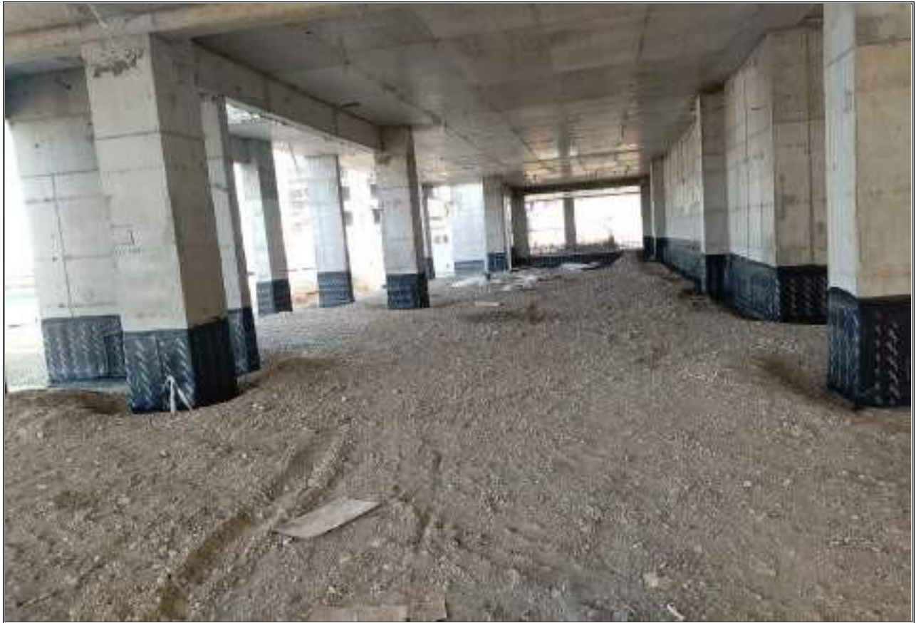
SUBSTRUCTURE WATERPROOFING CHEDI HOTEL RAS AL HADD – SUR
