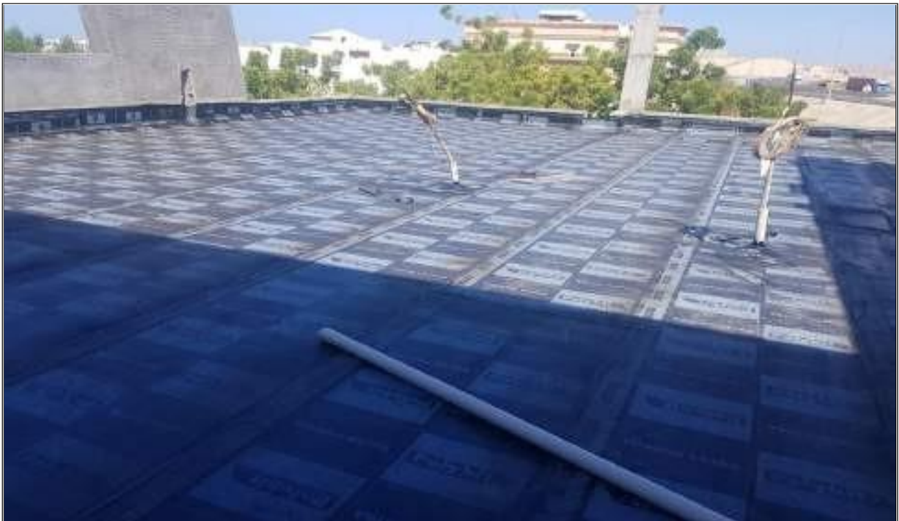
ROOF WATERPROOFING
