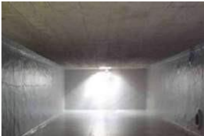
AL KHOUD COMPLEX SEWAGE TANK
