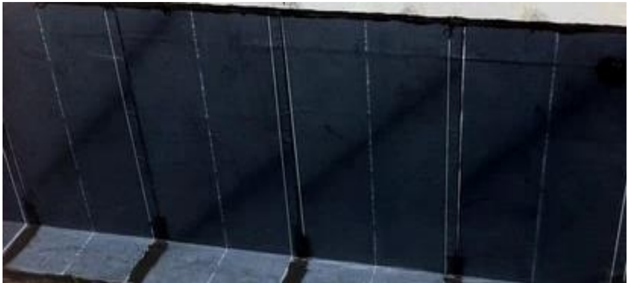
Self-Adhesive membrane work- STS for EES @ Rusayl
