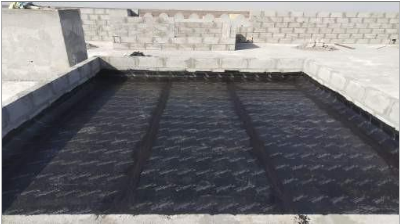
ROOF WATERPROOFING MOD – SOHAR
