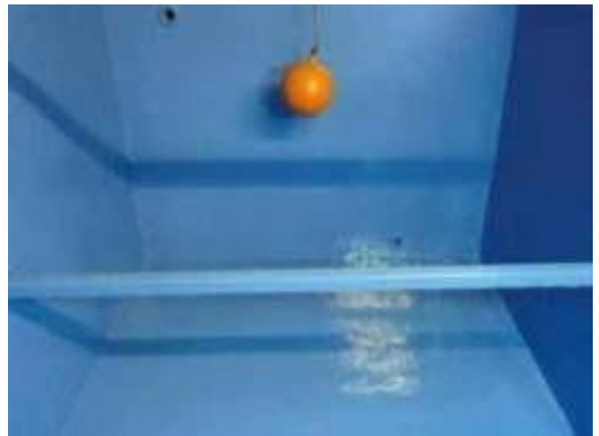
WATER TANK - GHALA
