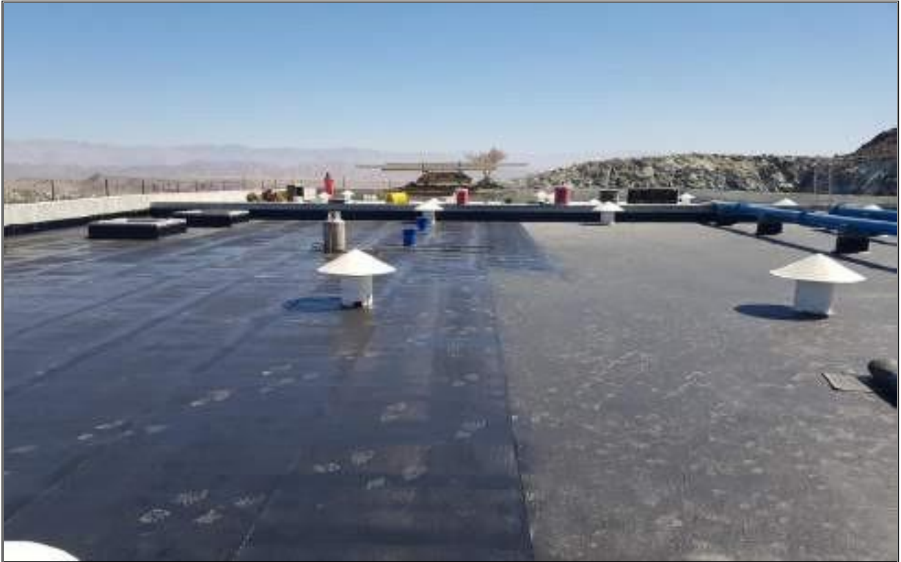
ROOF WATERPROOFING
