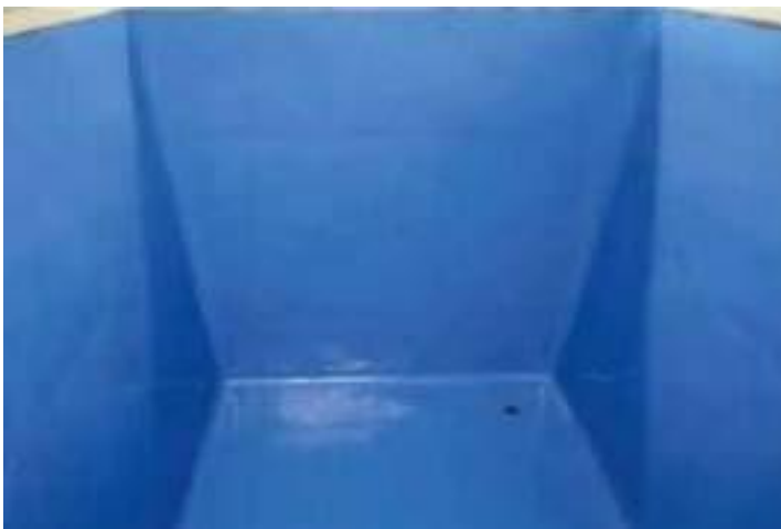
COMMERTIAL COMPLEX TANK – AL KHOUD
