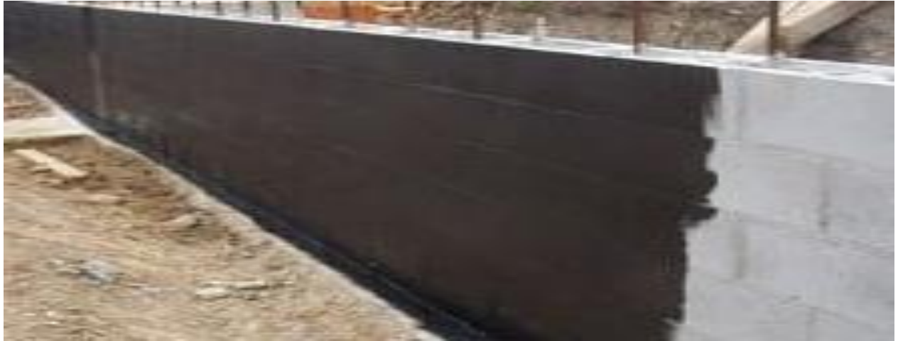
Self-Adhesive membrane work- STS for EES @ Rusayl
