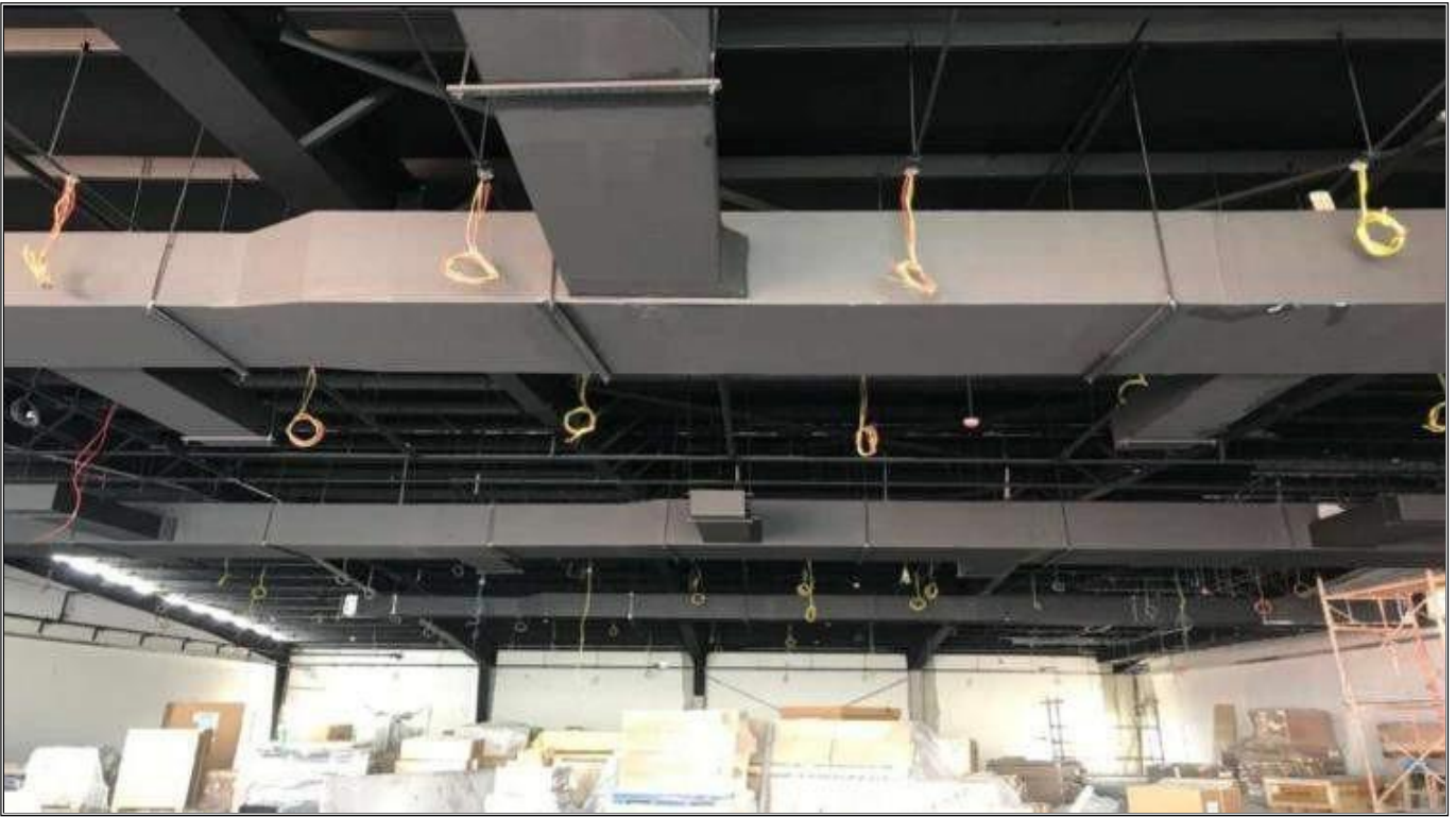
WAREHOUSE WORK - DUQM
