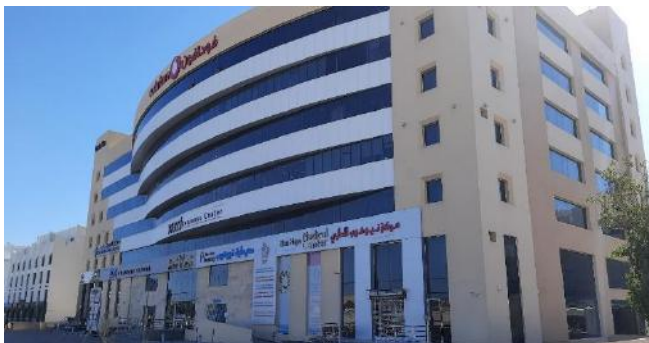
MAINTENANCES & RENOVATION WORK - CONSTRUCTION OF NEW HOPE HOSPITAL
