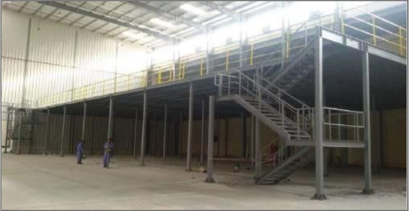
WAREHOUSE WORK – NIZWA
