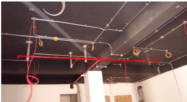
MAINTENANCES & RENOVATION WORK - NOVEC 1230 INSTALLATION AT NEW MAZDOON H.O AT FANJA
