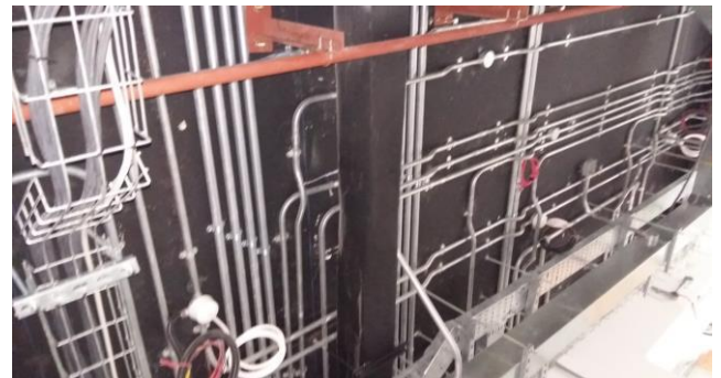
MAINTENANCES & RENOVATION WORK - ELECTRICAL CONDUITING & TRUCKING WORKS AT NBO H.O, AZAIBA
