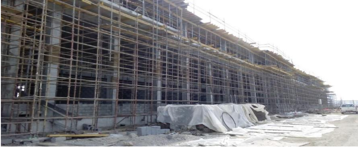
MEP WORKS @ SANDAN INDUSTRIAL CITY - HALBAN
