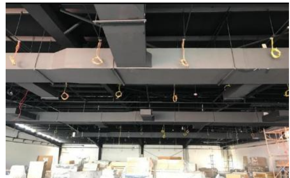
MAINTENANCES & RENOVATION WORK - WARE HOUSE AT DUQM
